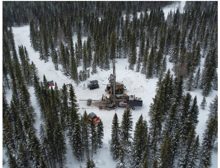
Aerial view of the active sonic drill during the Geotechnical and Hydrogeology Drilling Program. Several small drilling scopes were completed across the Crawford site this winter to help support and progress ongoing permitting and engineering.
